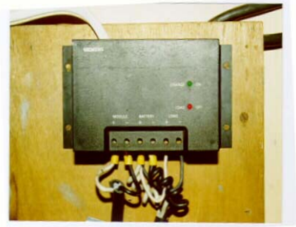
Illus. M PV module, battery and load connected to BCC
